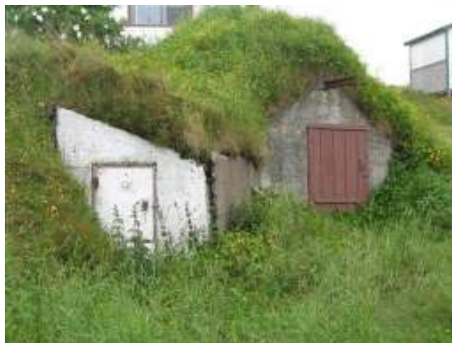
Root cellar, Port Rexton
